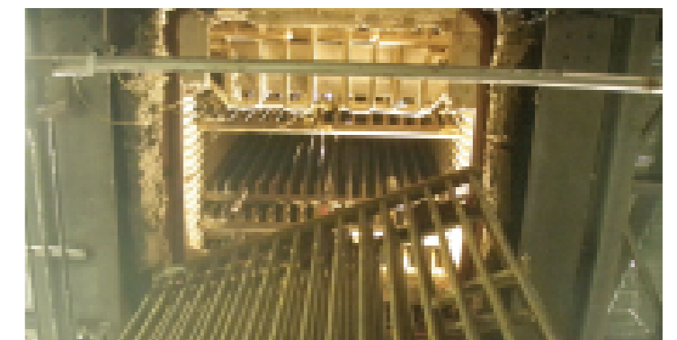
Working successfully in confined spaces.....
