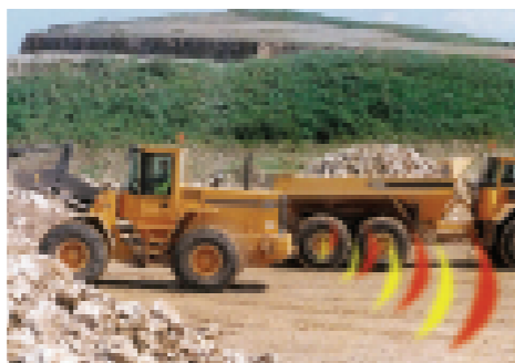
VMS Radar system
